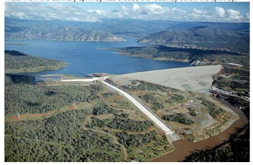
To lower the lake level, thus reducing flows and the potential for erosion at the top of the emergency spillway, DWR increased flows down the main spillway to 100,000 cubic feet per second from 55,000 cfs. This is the spillway that HydroWorld.com reported on Feb. 10 was damaged, when a cavity opened on the concrete due to erosion. DWR says current releases remain within the capacity of downstream channels.
